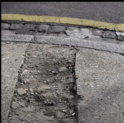
Water and Salt causes cementitious surfaces to corrode
