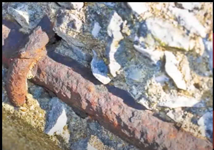
Rusted rebar swells to more than twice its size once corroded - causing damage to the concrete
